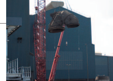
A crawler crane is used to install the diverting element of the cooling tower for Converter K 21.
